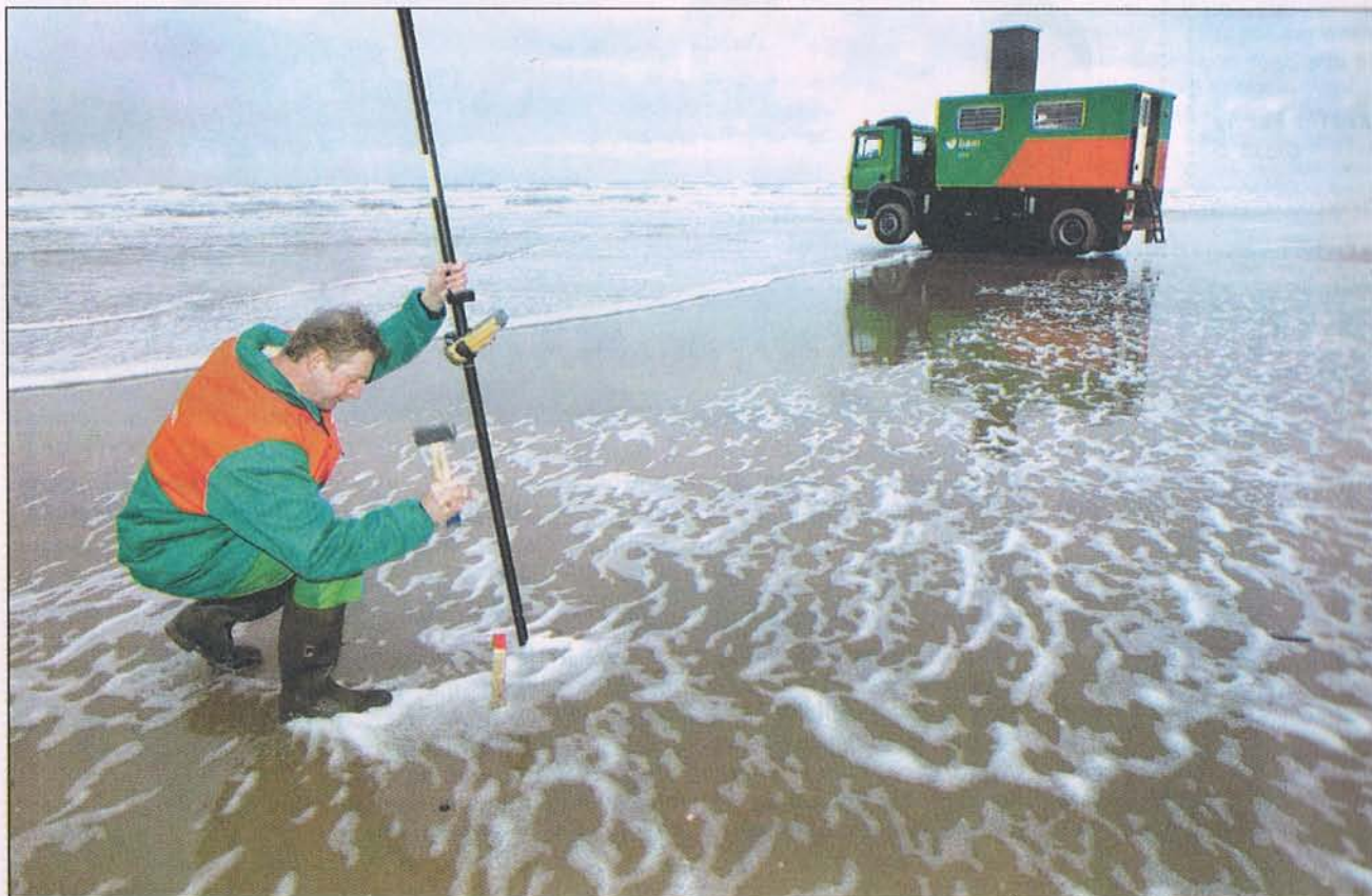
Eco-beach ... A meter determines where a special truck will place vertical drainage pipes in the beach at Egmond aan zee in the Netherlands last week. This new method to preserve the coast is being tested and is called Eco beach. It is an innovative system which ensures a wider and dryer beach because sand carried in by sea is stored better.
